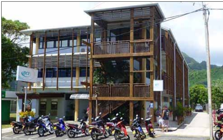
Thousands of offshore entities are headquartered on this building's third floor, which houses TrustNet's Cook Islands office. Photo: Alex Shprintsen
