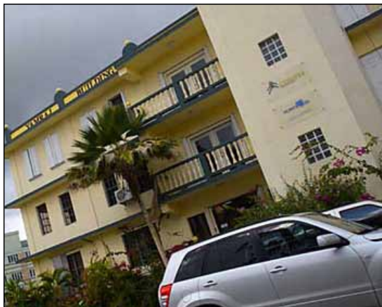
The BVI offices of offshore services company CTL. Photo: Alex Shprintsen
